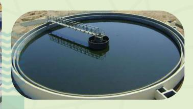
~Combined unit that performs both flocculation and clarification processes to remove suspended solids from wastewater.
