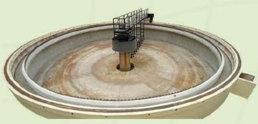
~ Settling tanks designed to separate solid particles from wastewater using gravity.
